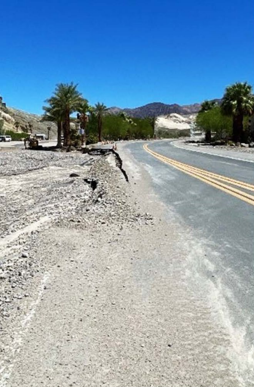
State Route 190 Inyo County
