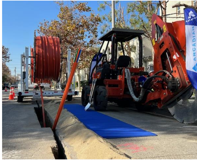
Figure 6: Microtrenching to install conduit
